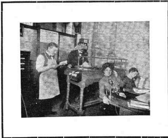
PART OF MAIN OFFICE.
